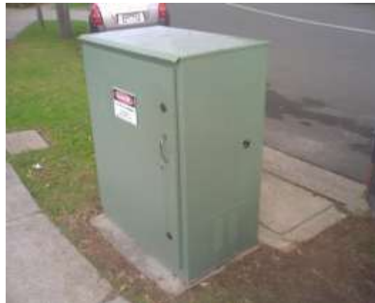
Figure 4. An example of the monitoring huts located at both the catchments. These huts contain the autosampling equipment required to conduct wet weather sampling at the catchments.
